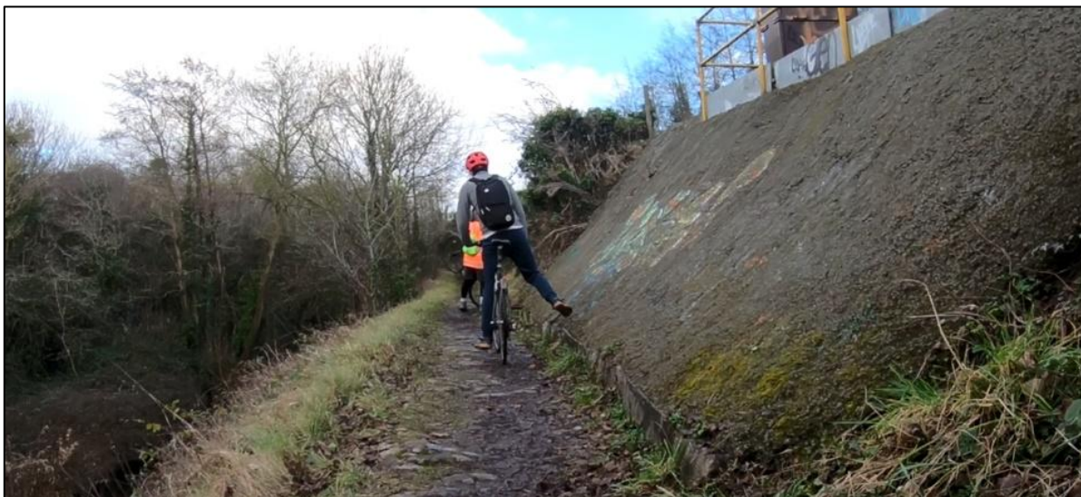
Figure 1-7 Pinch point between towpath and the railway signal
